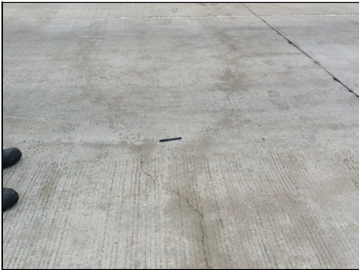
Unsealed cracks to Approach Slab @ Abutment 1.
