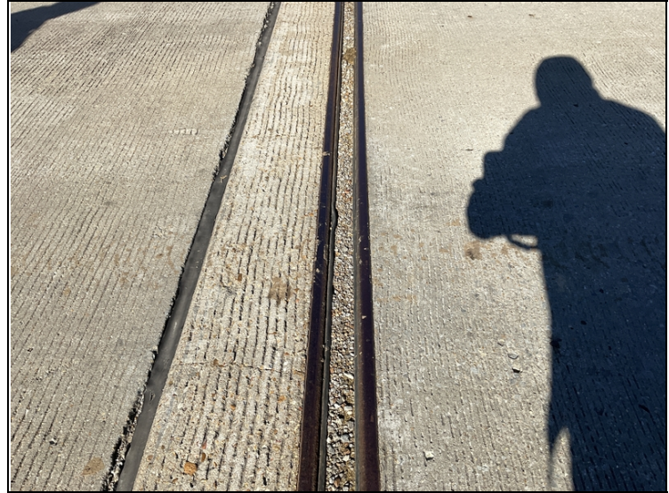
Debris impactation to compression joint seal @ Abutments 1 & 2. Abutment 1.
