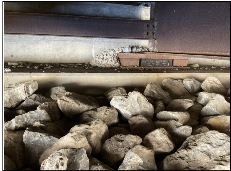
End of Girder 4 @ Abutment 2 Large concrete spill on cap, between bearing pad and backwall is restricting expansion.
