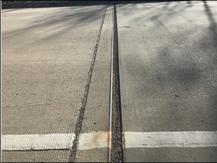
Debris in compression joint seal @ Abutment 1.
