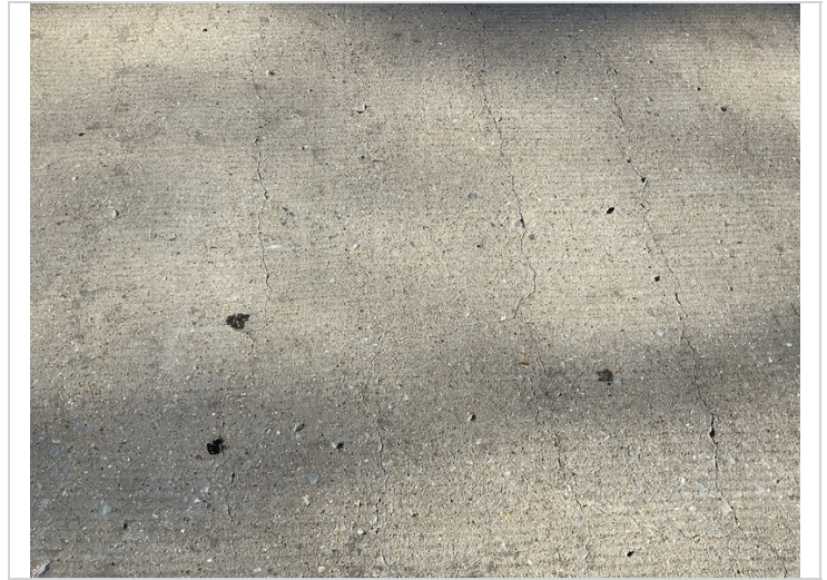
Typical cracks to deck @ all spans.
