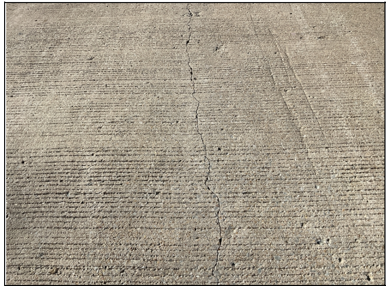
Approach Slabs @ Abutments 1 & 2 Several Transverse and Longitudinal unsealed cracks
