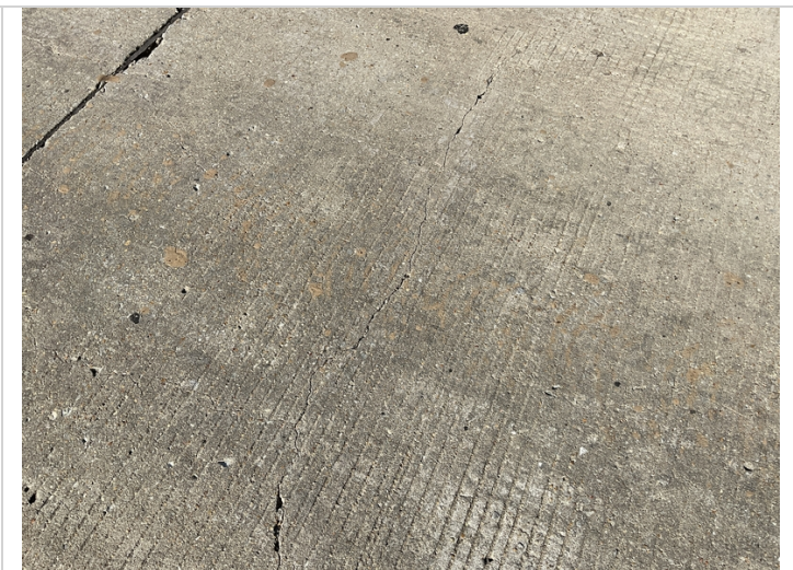
Typical cracks to approach slabs @ abutments 1 & 2.
