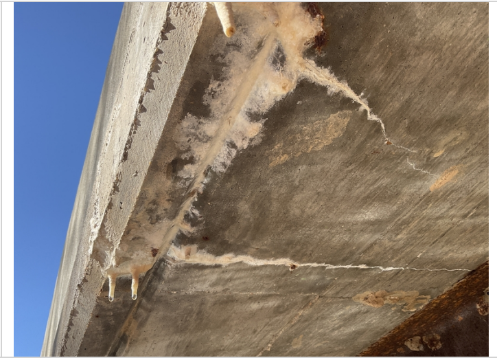
Typical efflor cracks to Lt & Rt overhangs.
