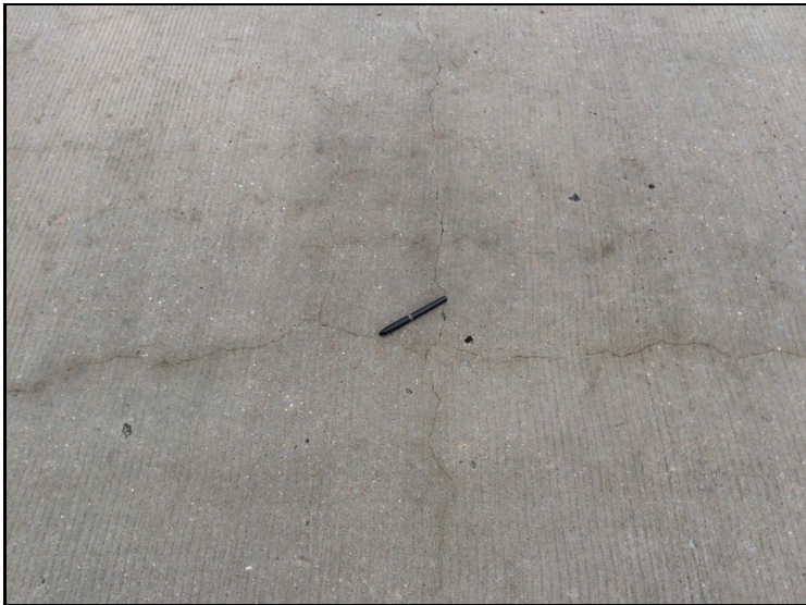
Several transverse and longitudinal unsealed cracks to all spans.
