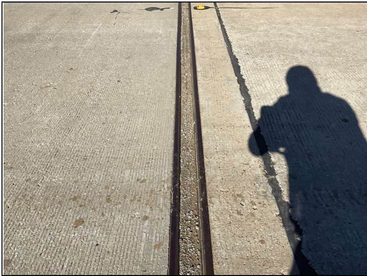
Debris impaction to compression joint seal @ Abutments 1 & 2. Abutment 2.
